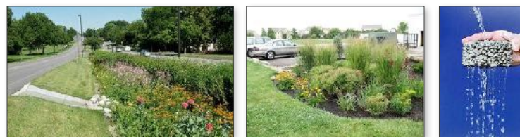
Bioswale, raingarden & permeable concrete
