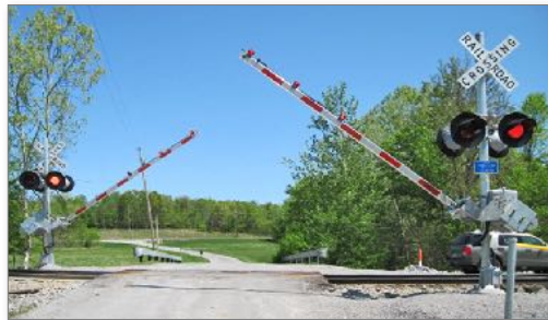
railroad crossing with automatic gates, cross buck signs and lights
